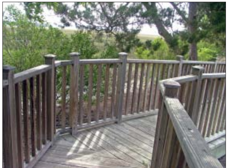
A broad ramp will make the first level of the new Alyea tower accessible to all.
